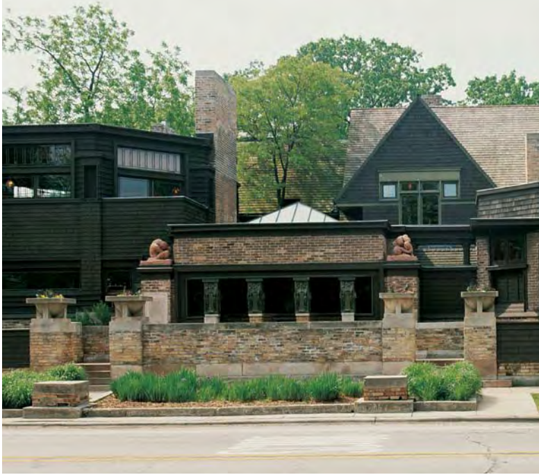
The Oak Park Home and Studio - Oak Park, Illinois - 1890-1909. Wright's own home and studio became an architectural laboratory during the nineteen years that he lived and worked there. Built in the same neighborhood as several of his other houses, it was a showroom of his ideas. In 1890 he placed lighting within a ceiling grille, creating the first use of what would be known as "indirect lighting."
