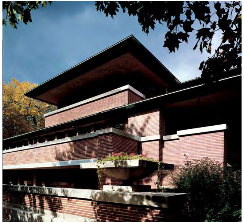
The Frederick Robie House - Chicago, Illinois - 1908. This house is often considered to be Wright's Prairie Era masterpiece. The client was an inventor and engineer who had specific requirements for the design. They include: a fireproof building, rooms without interruptions, all the daylight possible with shading and weather protection provided by overhanging eaves, the ability to see down the street to the neighbors with his own privacy ensured, and a walled yard to keep children from wandering off and getting lost.
